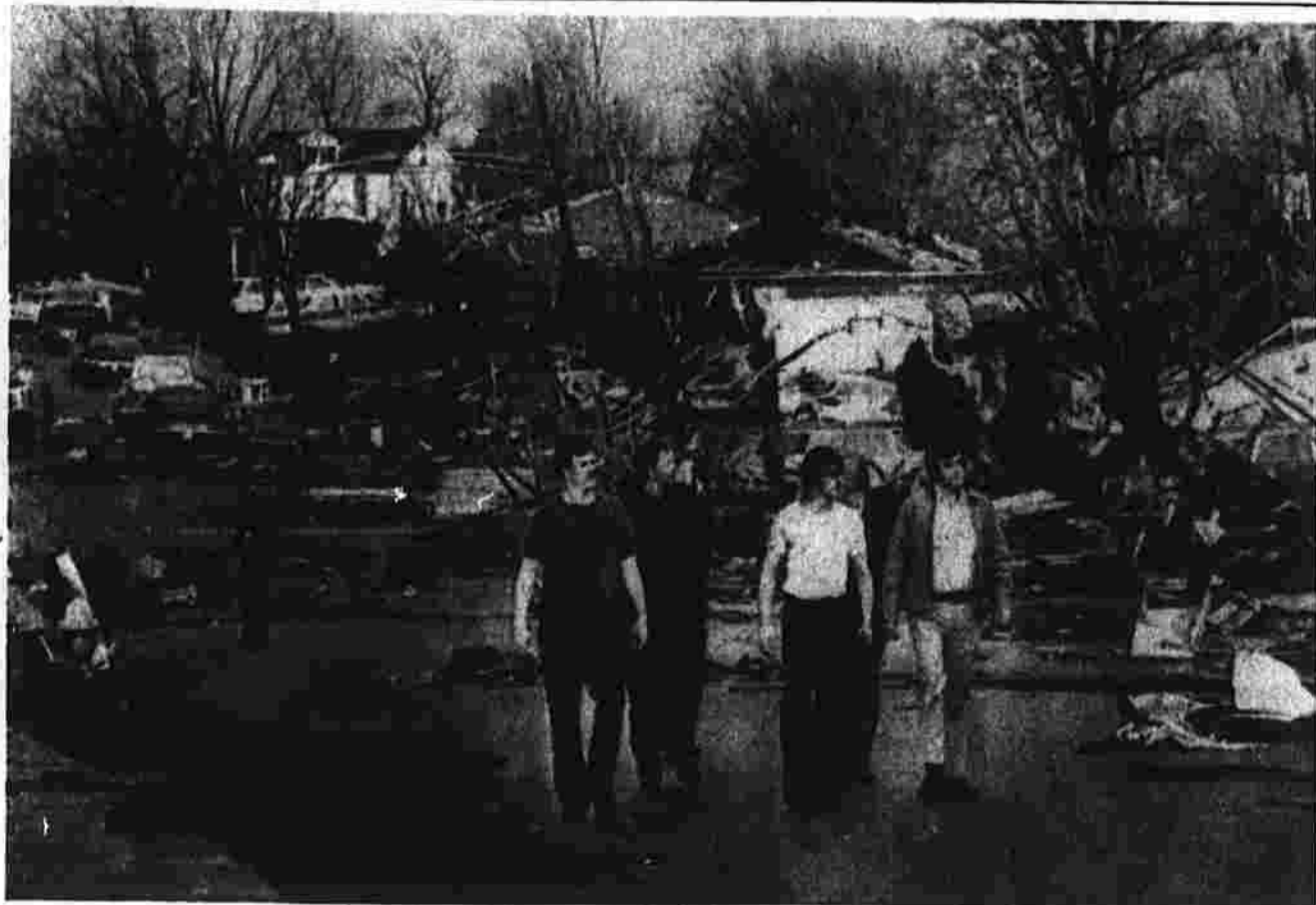
Most of the homes in this housing development in Xenia, Ohio, were ripped apart by the tornado which tore through the town, destroying about half the downtown area. (UPI Photo)
